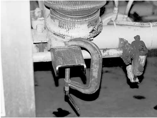
Figure 71: Temporarily holding beam extensions in place
