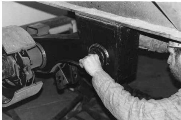
Figure 9: Installing new pivot connection hardware
